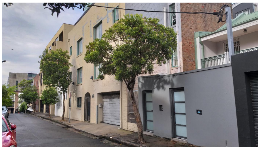
Properties opposite the site on Nimrod Street comprise mostly of rear elevations of low rise apartments and properties that front Victoria Street, garages and a car park.
